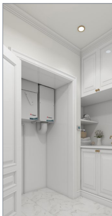
A MVHR cupboard installation
